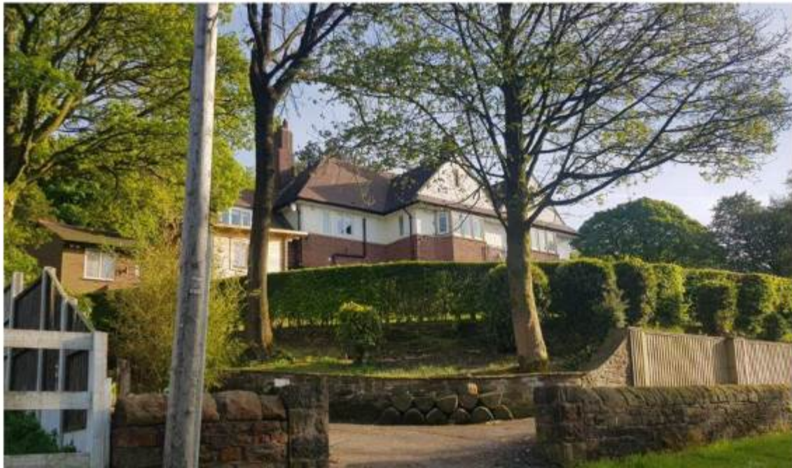
(2) The Braids from Woodgates Road [below]:
